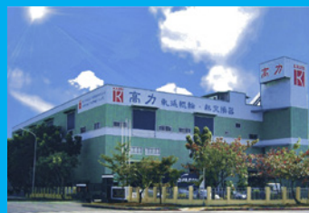
Kaohsiung Taiwan Plant
